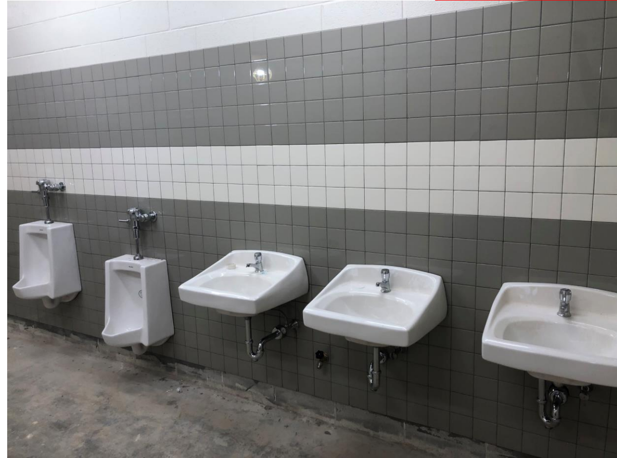
Plumbing Fixtures Installed in New Classroom Addition Restrooms
